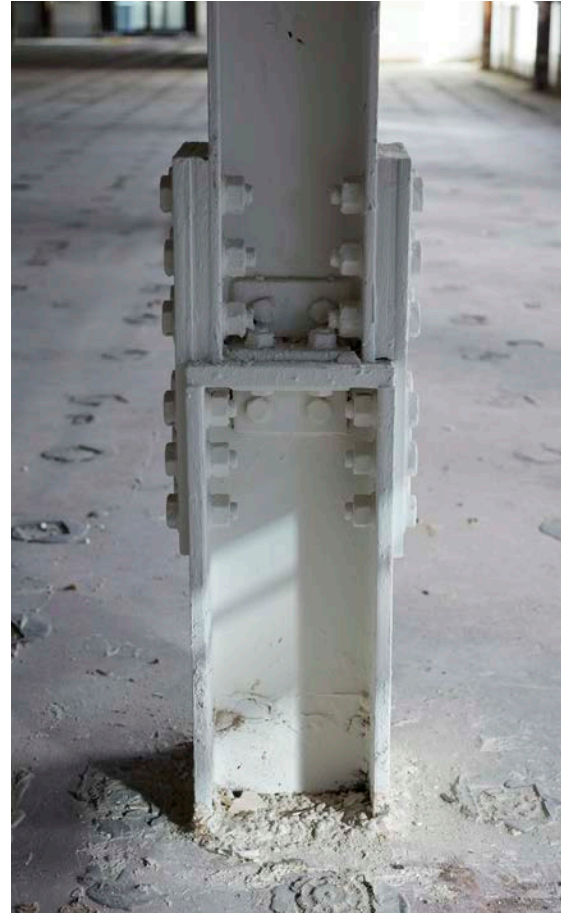
Column splice at Level 5
